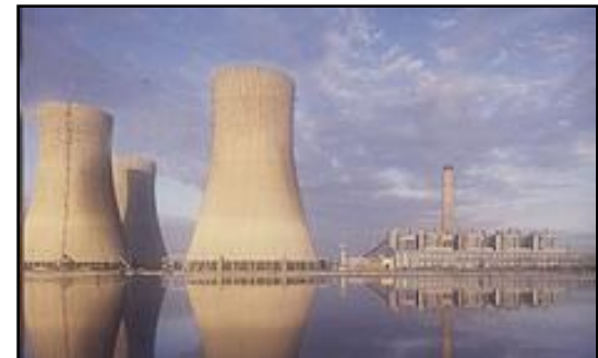
NTPC's Dadri Power Plant
