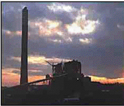
NTPC's 1000-MW Rihand Power Plant
