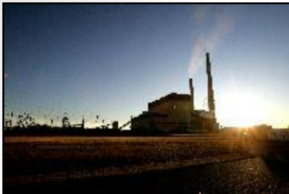
Alliant's Columbia Station
