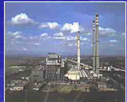
NTPC's 2000-MW Singrauli Power Station
