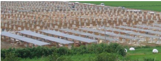
Installation of the solar modules commences
