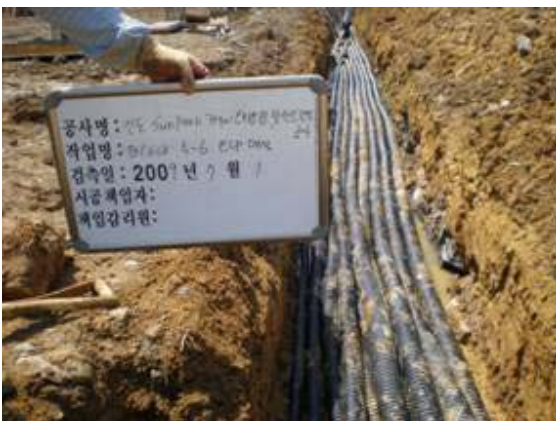
Installation of the LV cabling
