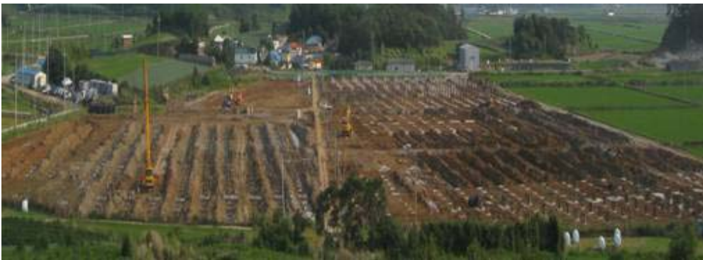
Panoramic view of the project site midway through construction (mid Jul-09)
