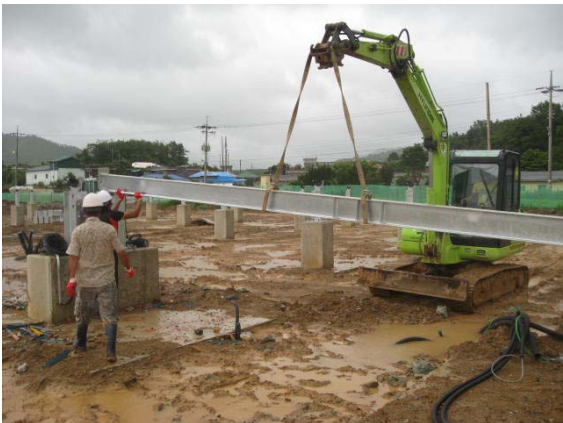
Installation of the base components of the tracking system
