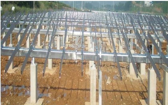
Installation of the module support components of the tracking system
