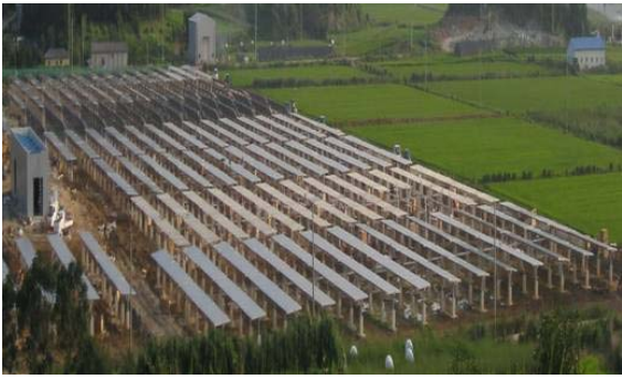
Substation under construction
