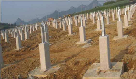
Installation of tracker steel posts on the concrete pillars
