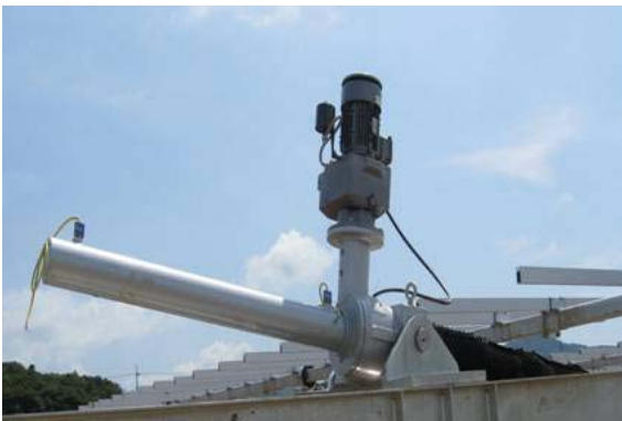
Installation of the Tracker Drive Units
