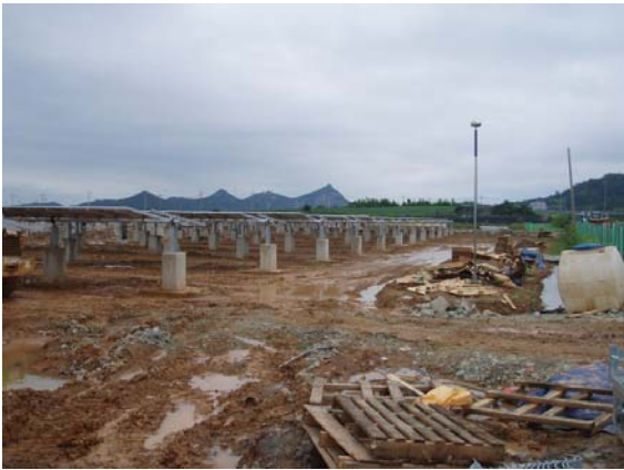
Installation of the solar modules
