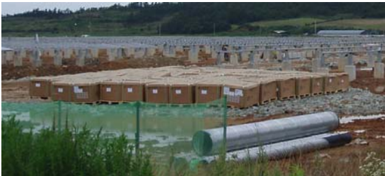
Delivery of the solar modules to site
