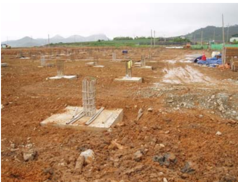
Installation of foundations and pillars to support the tracking system
