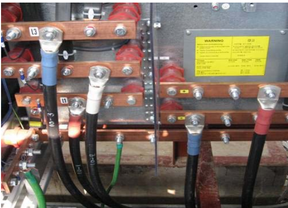
Inverter Connection (380VAC connection)
