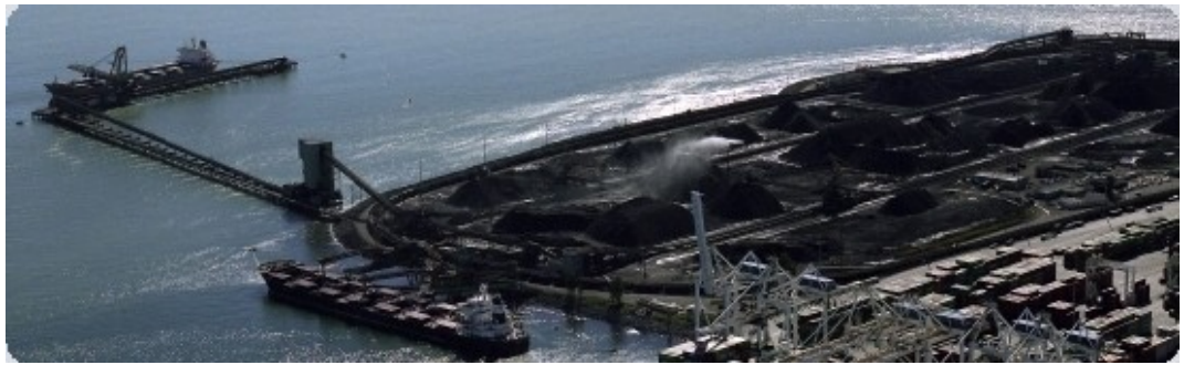
Westshore Terminals located at Roberts Bank, Delta, Canada.
