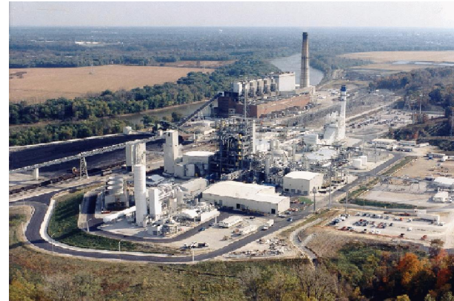
Wabash 252MW, US
