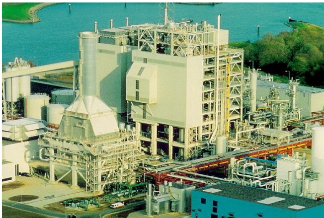
Buggenum 250MW, The Netherlands
