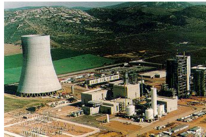
Puertollano 300MW, Spain
